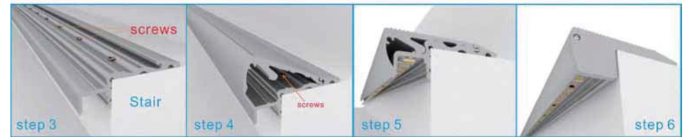
Step 3: Separate two part of profile, Step 4: Slide part A to part B, fixed Part B with screw. Step 5: profile with strip Step 6: fixed end cap with screw.
