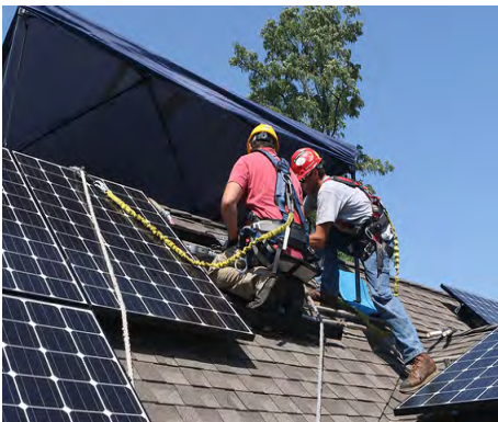
33KW Grid Power Station
