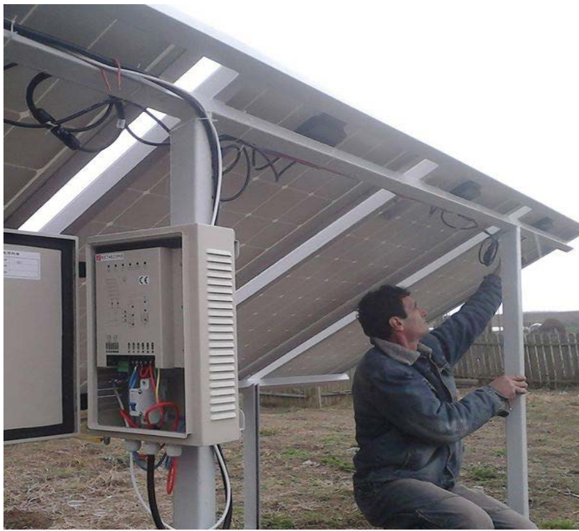
4SP8-7A Solar Water Pump 9pcs 235Wp solar panel 110V MPPT controller
