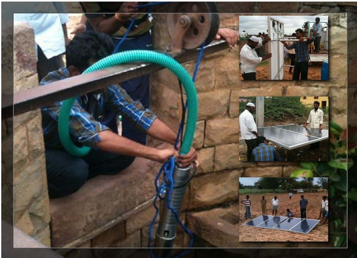
4SP3-12A Solar Water Pump 8pcs 180Wp solar panel 110V MPPT controller
