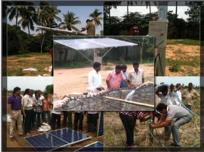
4SP2-9A Solar Water Pump 4pcs 180Wp solar panel 48V MPPT controller
